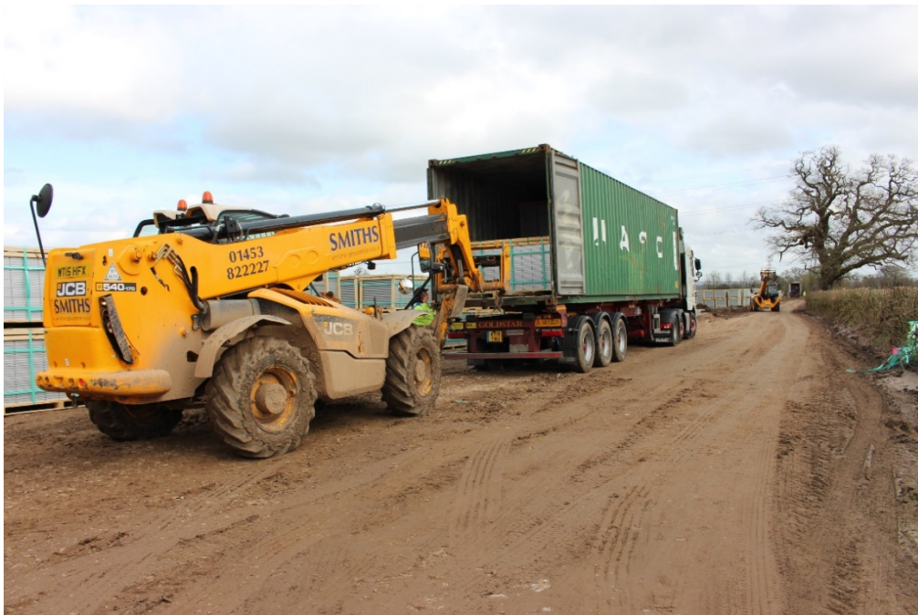
Plate 7: Delivery of construction materials, plant and equipment to Site
