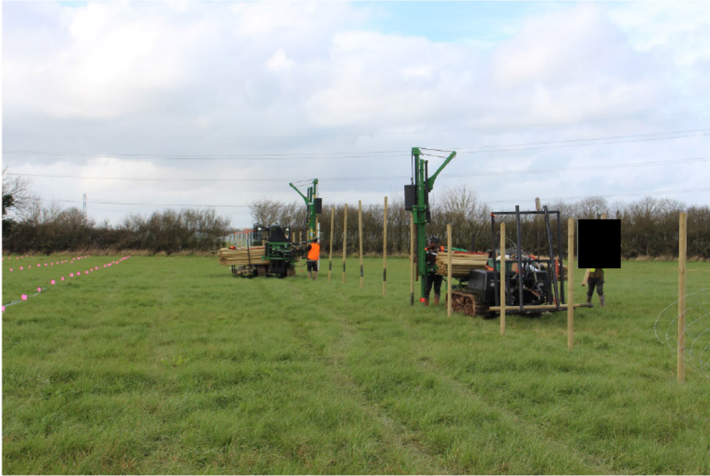
Plate 8: Establishment of Site fencing
