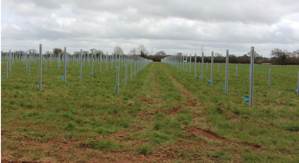
Plate 11b: Installation of Mounting Structures (2 of 4)
