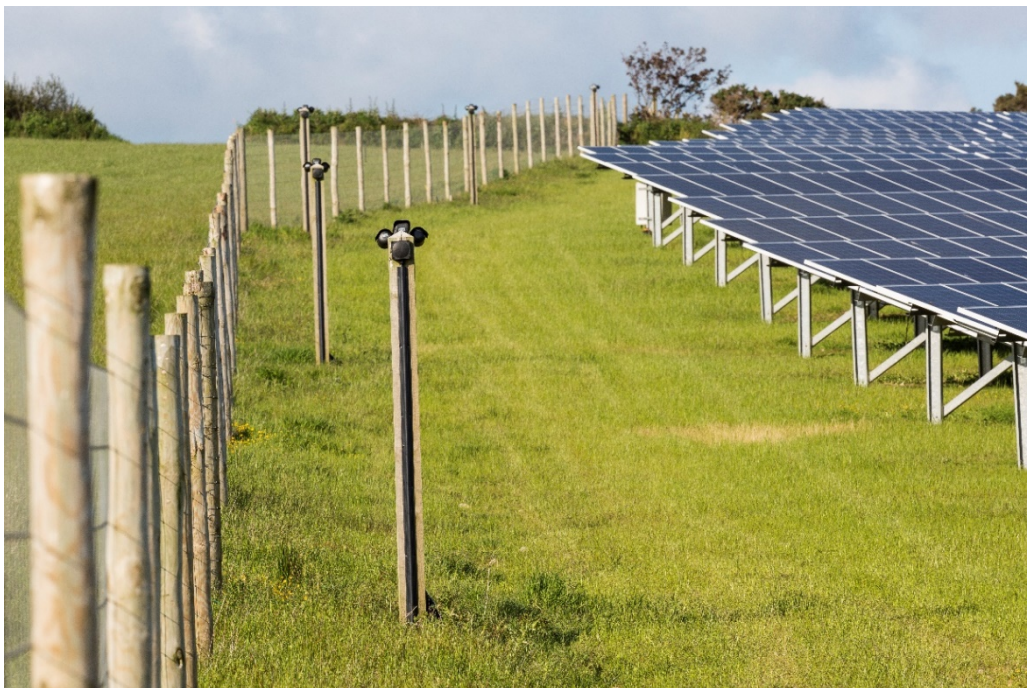
Plate 5: Example of security fencing and monitoring cameras
