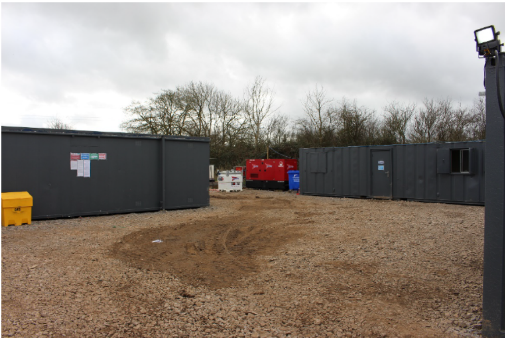
Plate 9: Establishment of the temporary construction compound(s)
