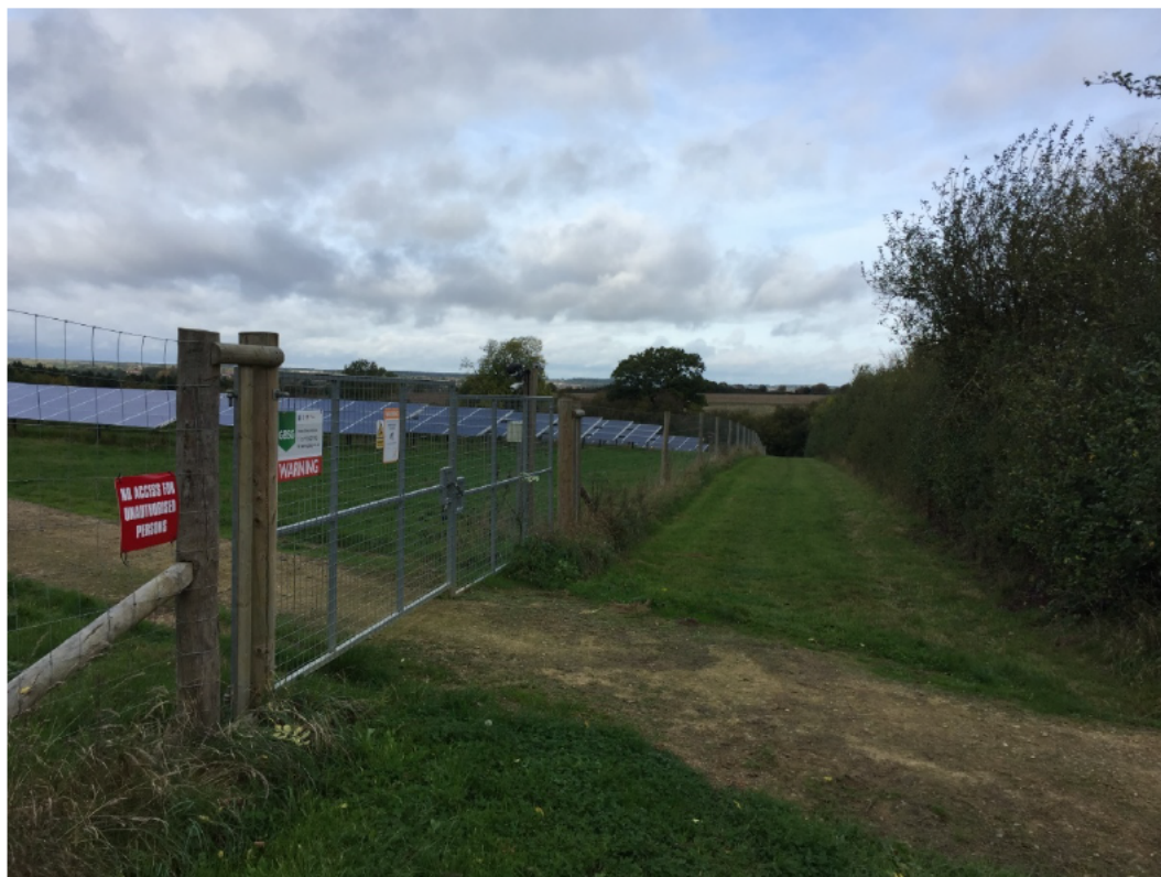
Plate 6 – Example image of a security fence, access gate, CCTV camera, internal access track.
